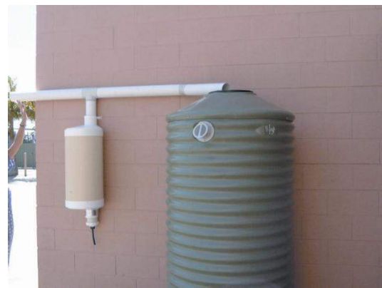
Typical Wall Mounted First Flush Installation (Applicable to Product Codes: 8121-1, 8119-5 & 8118-8)
