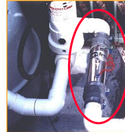
Care Free installed on Swimming Pool Filter/Pump system
