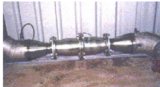
100mm unit installed on an Effluent Treatment Plan
