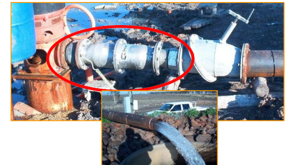
Installed on Irrigation system
