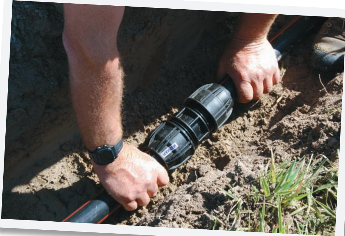
Hansen Medium Density Coupling (HMDC) in use
